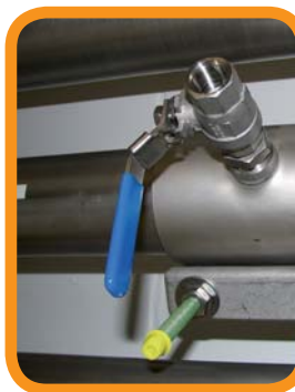
B Spot drilling collar
