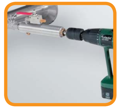
Drilling under pressure
